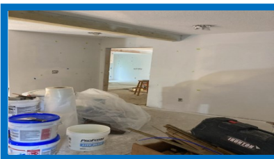
Working on walls and ceiling
