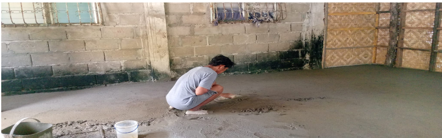
They mixed and finished the cement for the floor.
